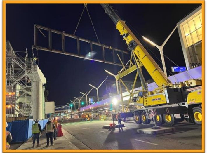
Top: A section of steel is lifted into place overnight
