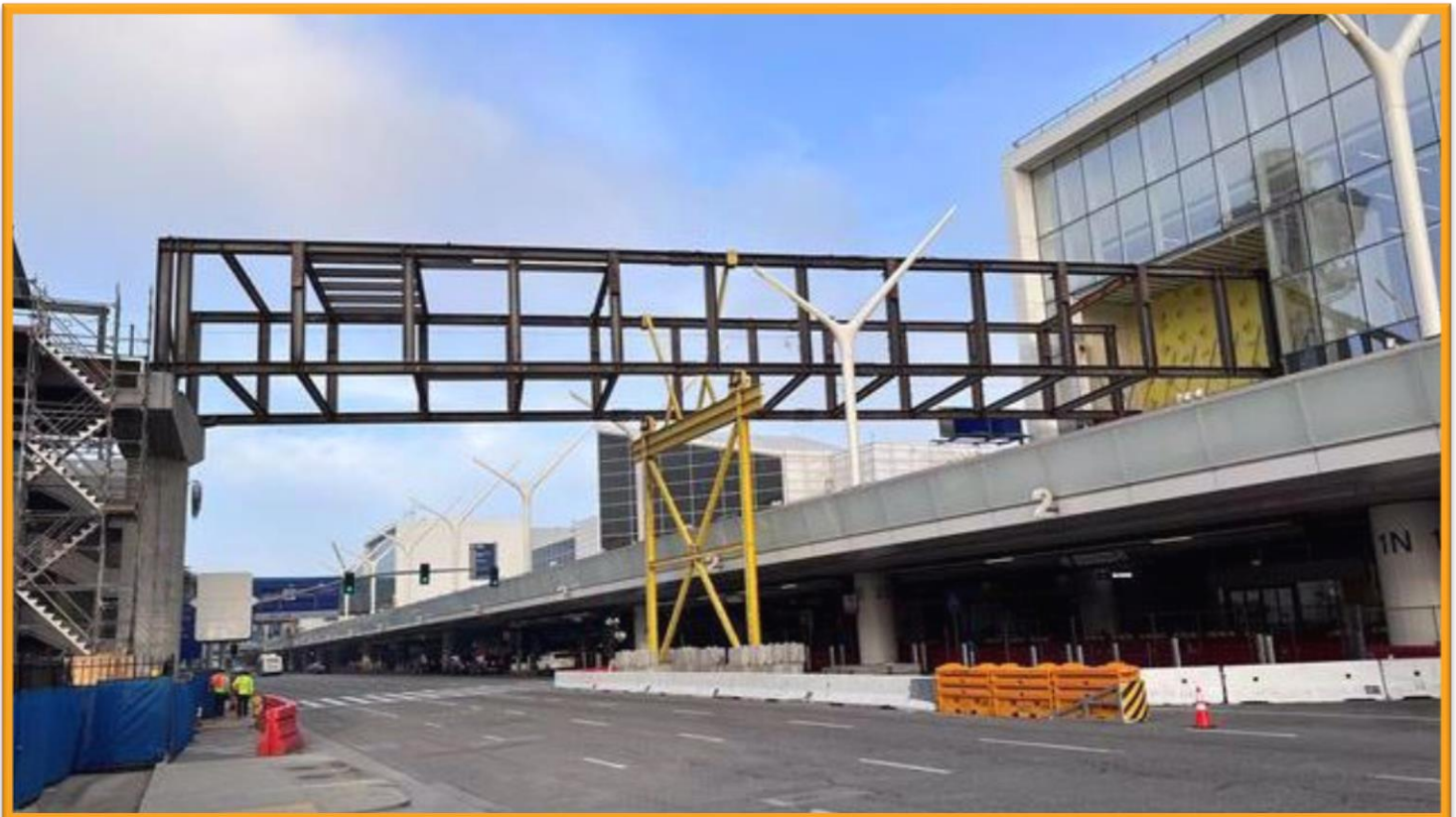
Bottom: Completed steel structure of the pedestrian bridge
