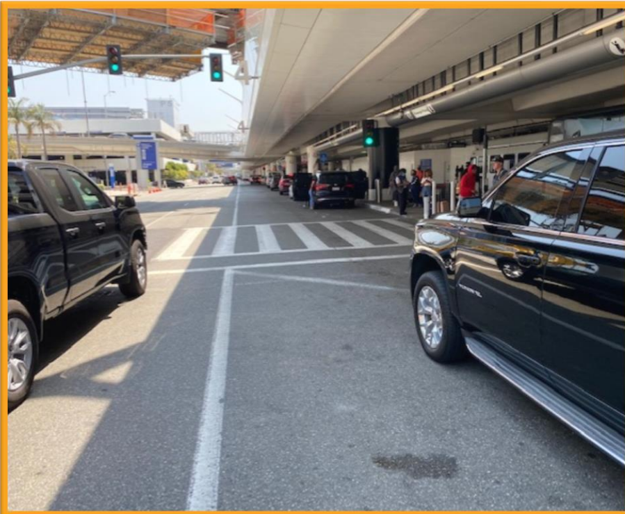
Shoring tower removed & lanes re-opened July 2021
