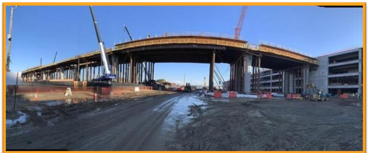
APM guideway connecting with ConRAC Facility (building at far right)
