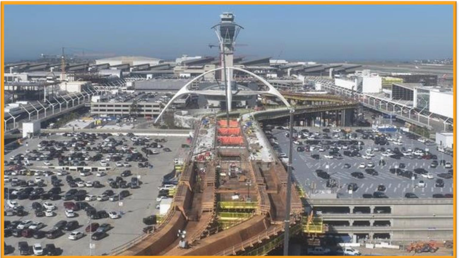
APM falsework removal at CTA's East Station
