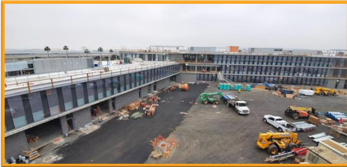
Ongoing construction at the new APF
