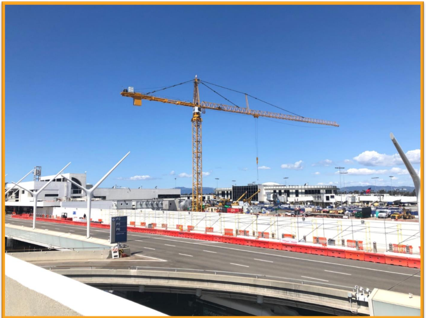
Departures Level construction between Terminals 2 & 3 (roadway)
