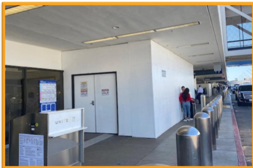
Terminal 7 Construction Barricades
