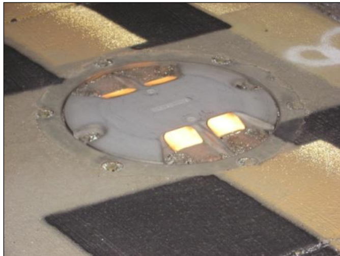
Flush-mounted Runway Light Fixture
