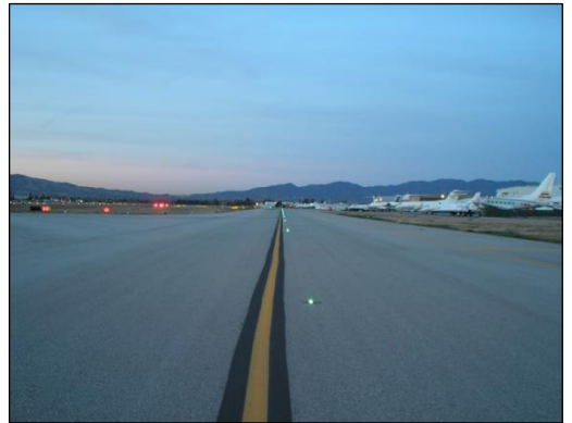
Taxiway Centerline Lights
