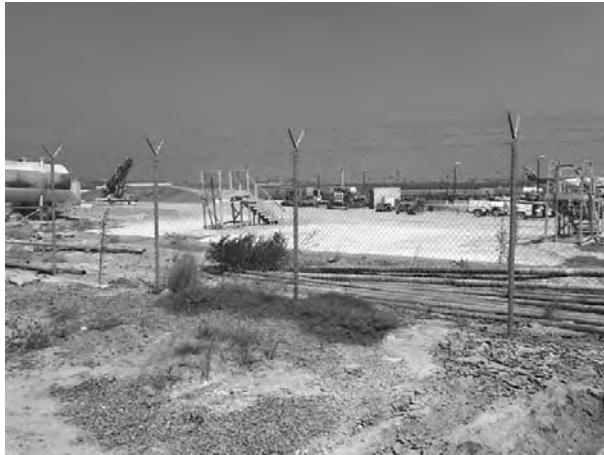
Representative site photograph depicting disturbed/developed areas in the northwestern portion of the proposed staging area.
