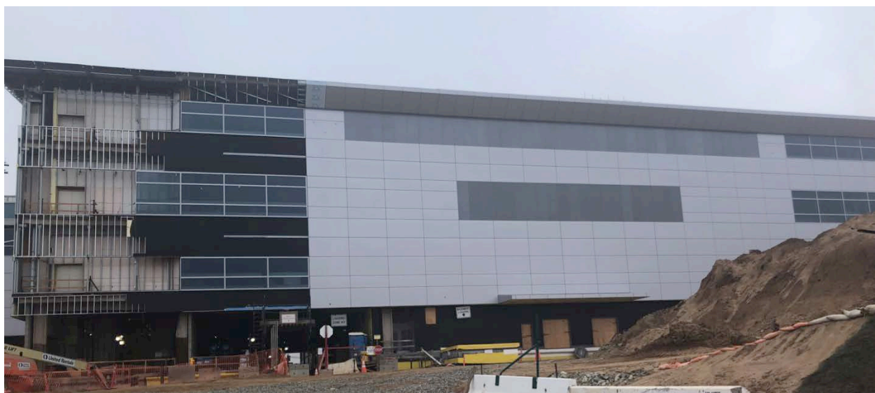
Figure 1-1 – Midfield Satellite Concourse North Project Progress
