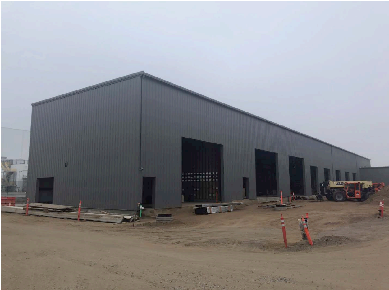
Figure 1-3 –WAMA Delta GSE Facility Project Construction Status
