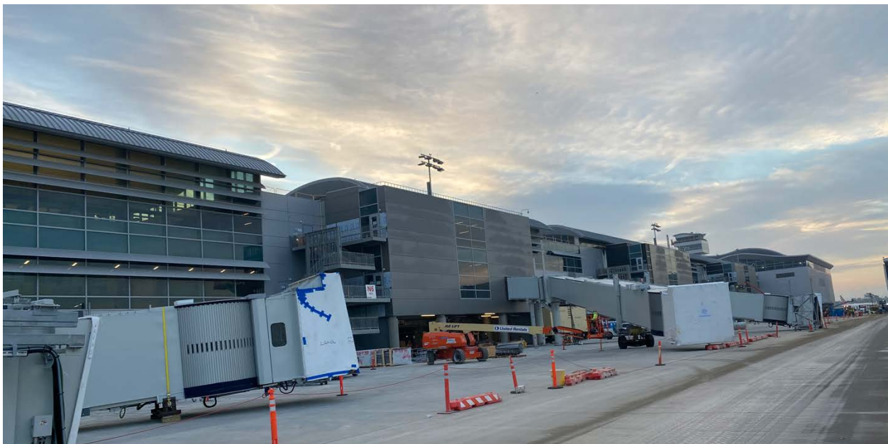
Figure 1-1 – Midfield Satellite Concourse North Project Progress
