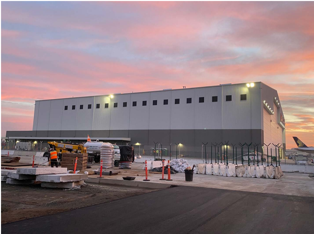
Figure 1-2 – WAMA Delta Hangar Project Construction Status
