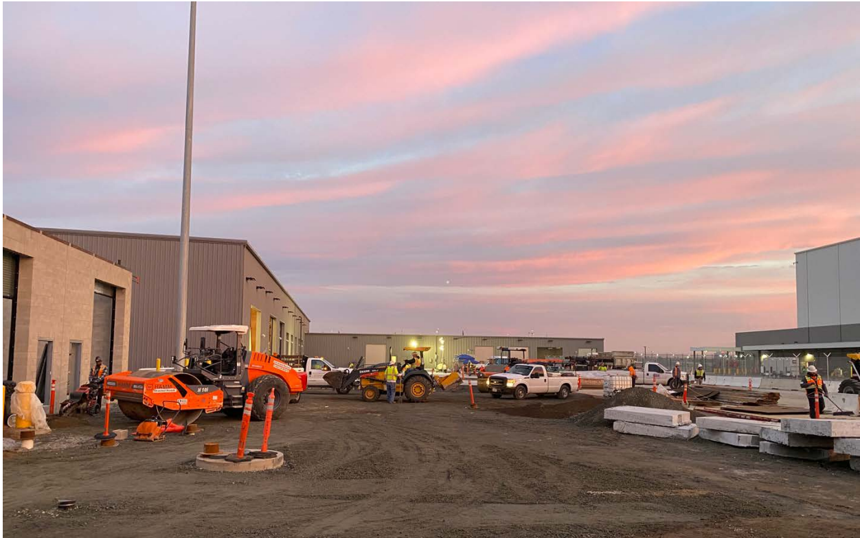
Figure 1-3 –WAMA Delta GSE Facility Project Construction Status
